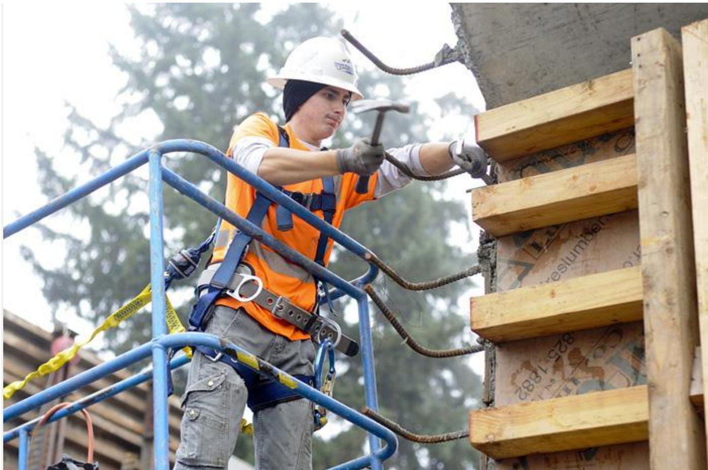
David Oancea, an apprentice laborer with Cascade Bridge and student at the Northwest College of Construction, strips concrete forms from a support column while working on an on-ramp project on I-205 in Vancouver, Wash.
